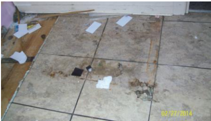
Hole in floor
